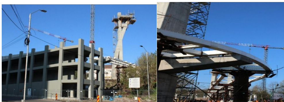
Figure 5. Stages of project implementation - Access to George Bacovia University
